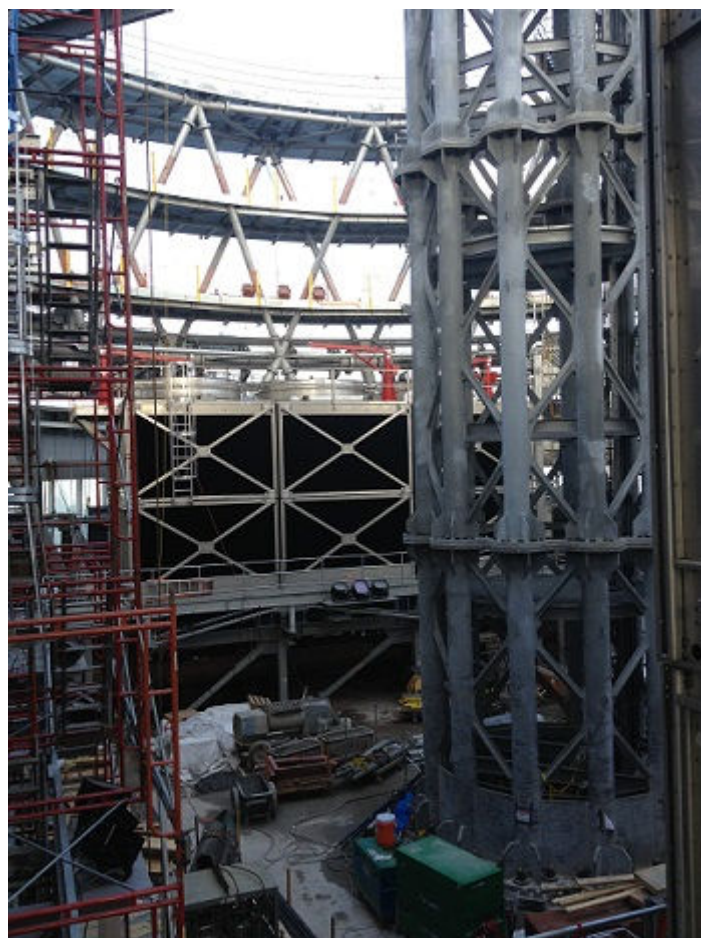
A view down onto the roof well. The base of the steel spire is at right. Master TV and FM antennas would be mounted on the spire; smaller systems like STLs, ENG, RPU and cameras will go on one of the three communication rings visible near the top center.
